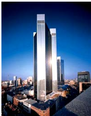
Compressive Strength 110 N/mm 2 186 m, BfG Bank, Frankfurt, Germany
