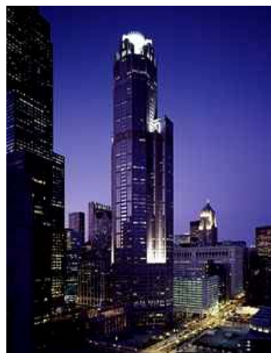
Compression Strength >80 N/mm 2 293 m, South Wacker Drive, Chicago, USA
