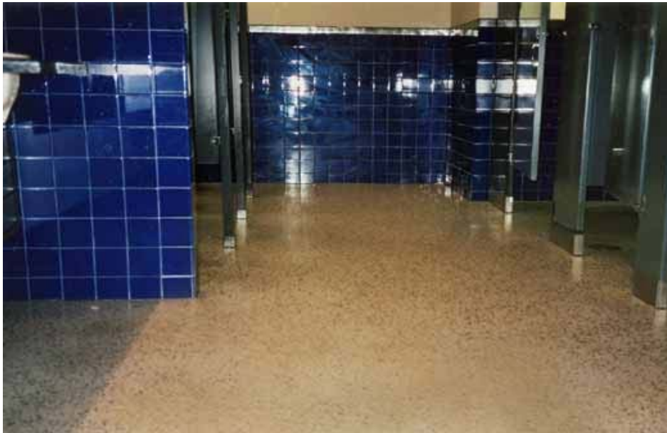
“Epo Bond SL 3” install at Hotel Toilet/Bath Room Floors
