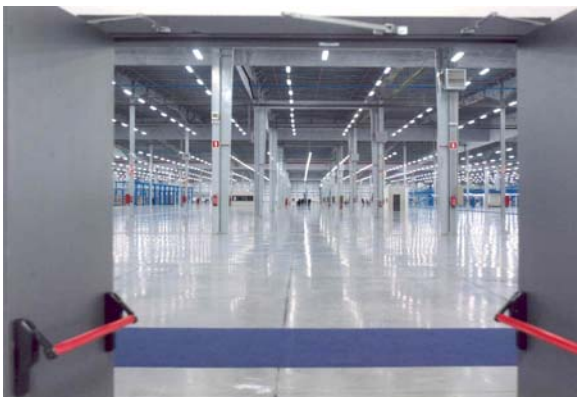
Epo Bond Water SL2#ZARA, Zaragoza, Spain
