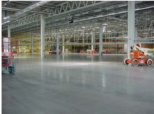
Epo Bond Water SL2#SAAB, Trollhattan, Sweden
