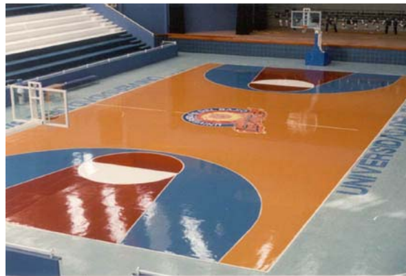
PUR Guard SF, Sport Floor Install on Indoor
