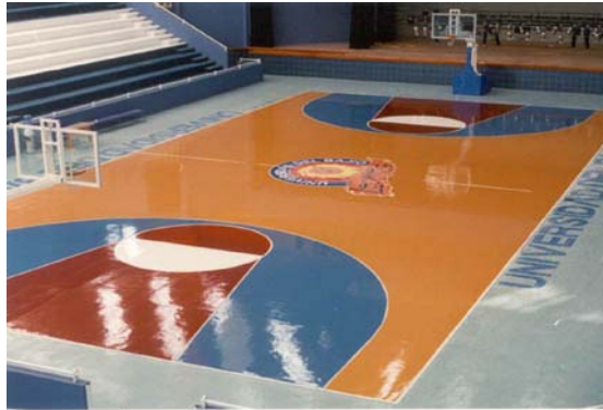
PUR Guard SR 100, Install on Indoor Multi Purpose Hall
