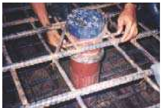
Installing around pipes
