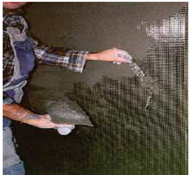
Install on Build Mesh CF 30020 on Wall
