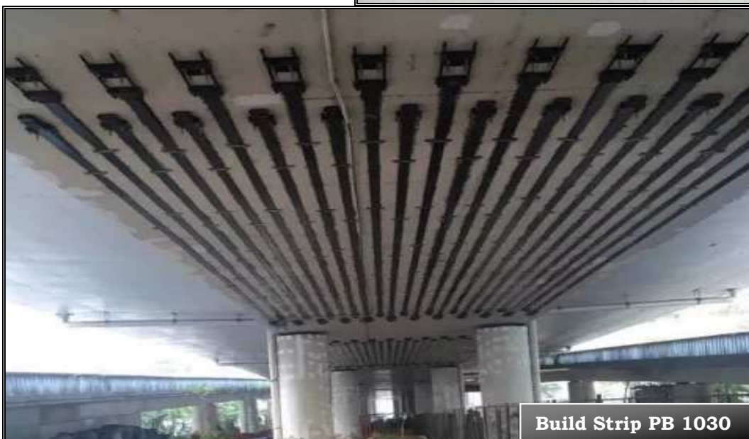
Build Strip PB 1030, install on under Bridges Deck
