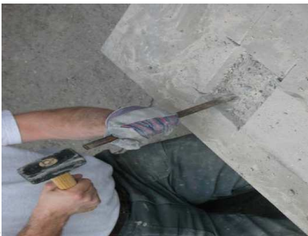
03 Maximal depth of cut 25mm
