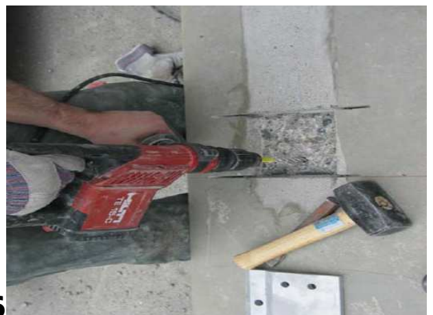
04 Complete the mill-cuts on all sides, but don't cut over the markings on face side
