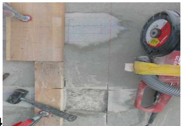
02 First-cut on face side with diamond blade
