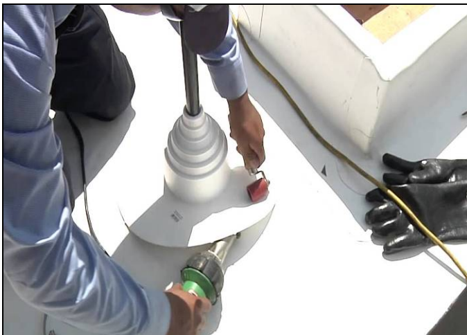
Install of Roof Gard SA for Roof Downpipe
