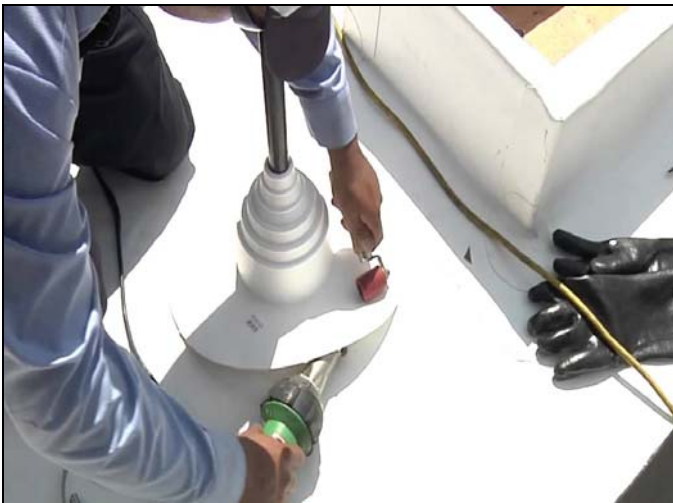
Install of Roof Seal PVC for Roof Downpipe
