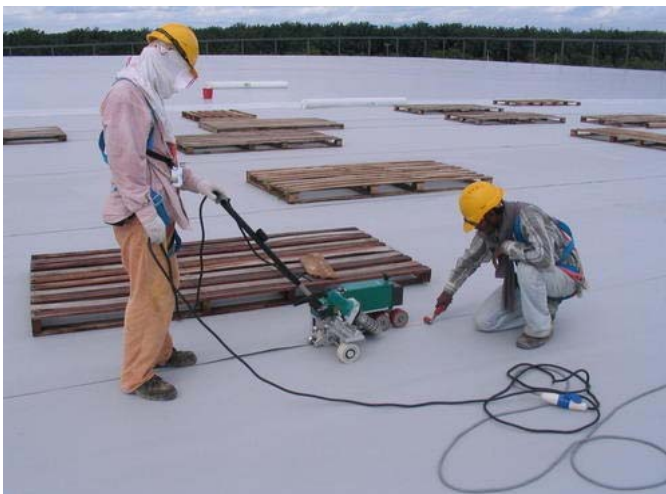
Roof Seal PVC 18P, 1.80mm thick for Expose Roof Slab
