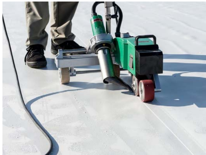
Welded Machine Laying Installation Overlap
