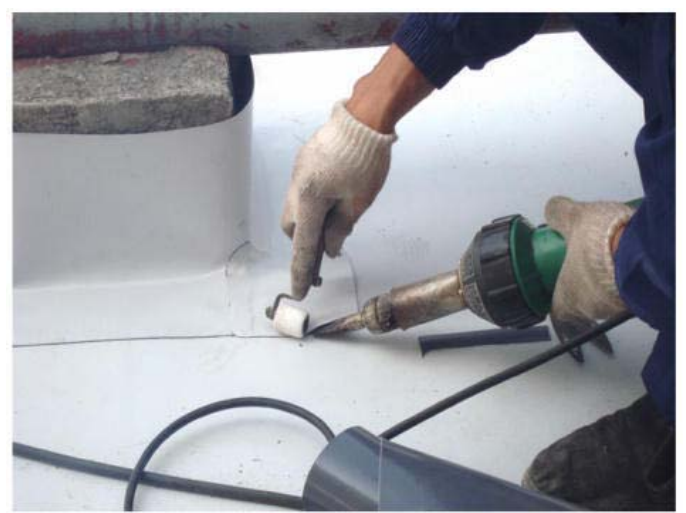
Method of Installation for Side Skirting
