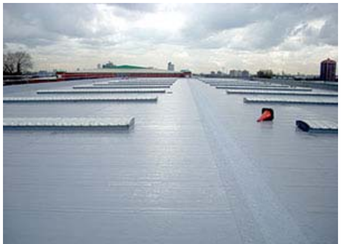
Roof Seal PVC 18P, 1.80mm thick for Expose Roof Slab
