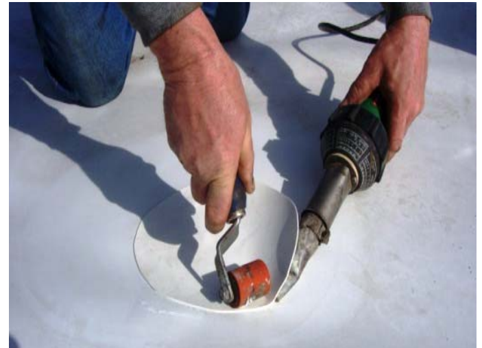
Method of Installation for Downpipe Hole
