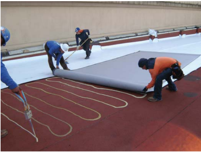
Applied of Epoxy Primer and Adhesive
