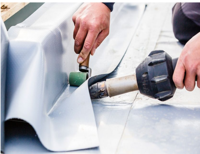
Method of Installation for Side Skirting
