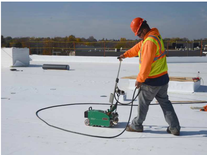
Roof Seal TPO 20P, 2.00mm thick for Expose Roof Slab
