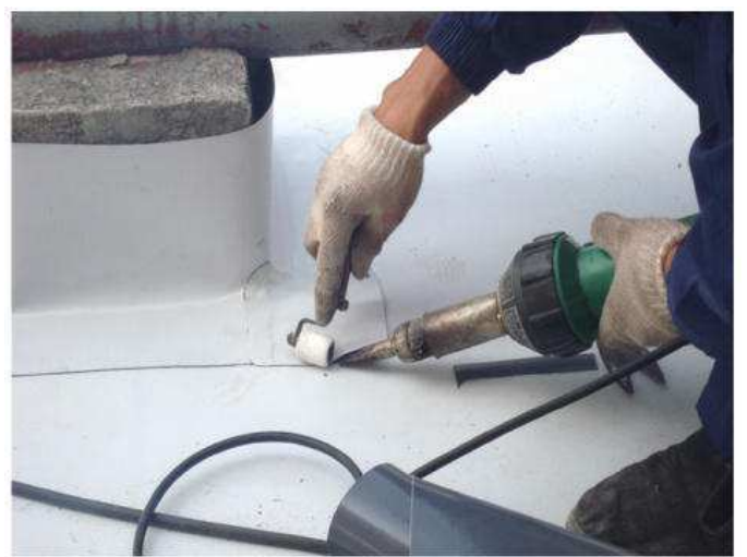
Method of Installation for Side Skirting
