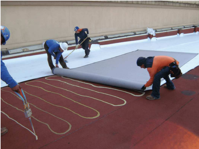
Applied of Epoxy Primer and Adhesive
