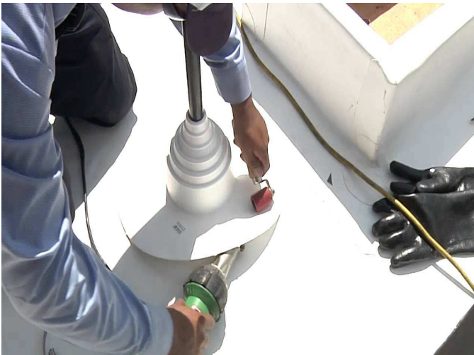
Install of Roof Seal TPO for Roof Downpipe
