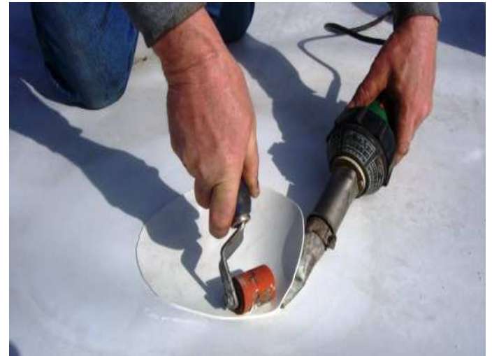
Method of Installation for Downpipe Hole
