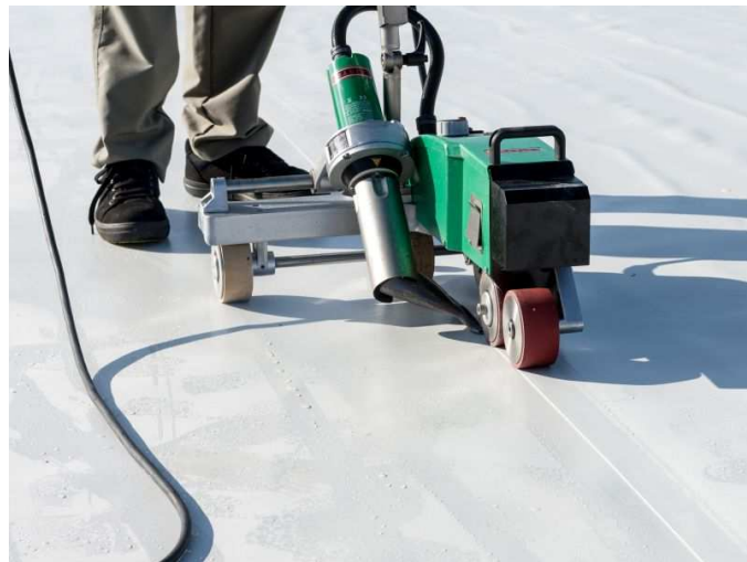
Welded Machine Laying Installation Overlap
