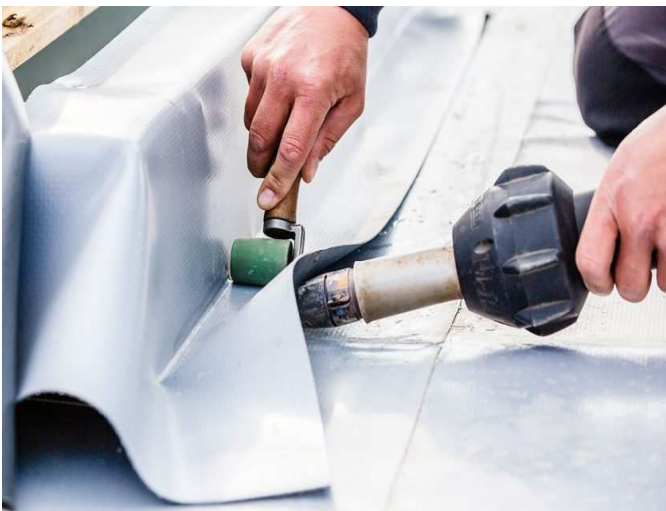
Method of Installation for Side Skirting
